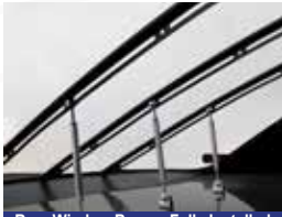
Rear Window Braces Fully Installed
