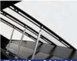
Windshield Braces Fully Installed
